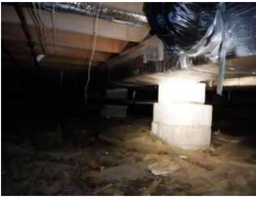
Photo X-52 Main Beam Support
