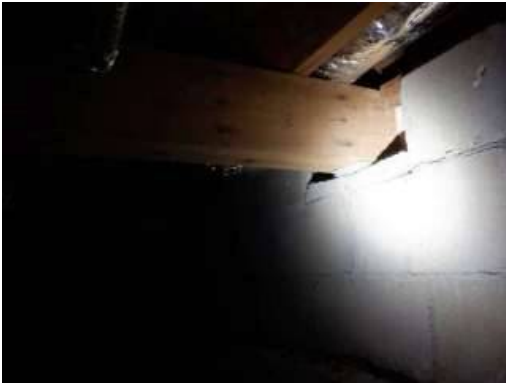
Photo 19-3 Main Beam in Crawl Space.
